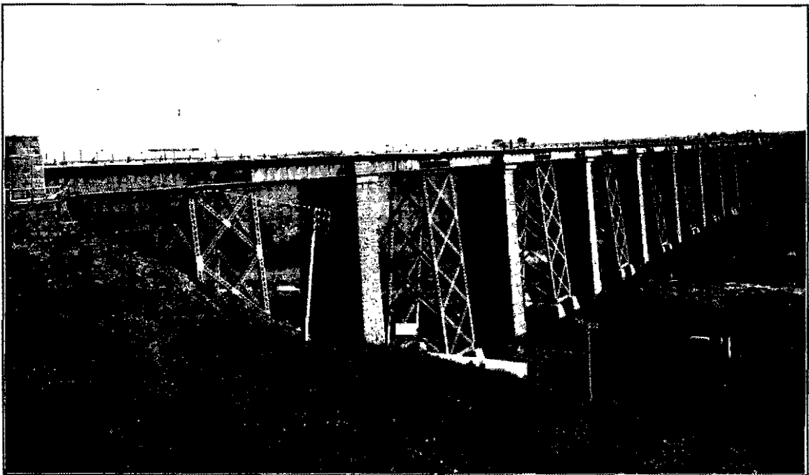
VIADUCT AS RENEWED TO CARRY LOCOMOTIVES OF 160 TONS WEIGHT.
